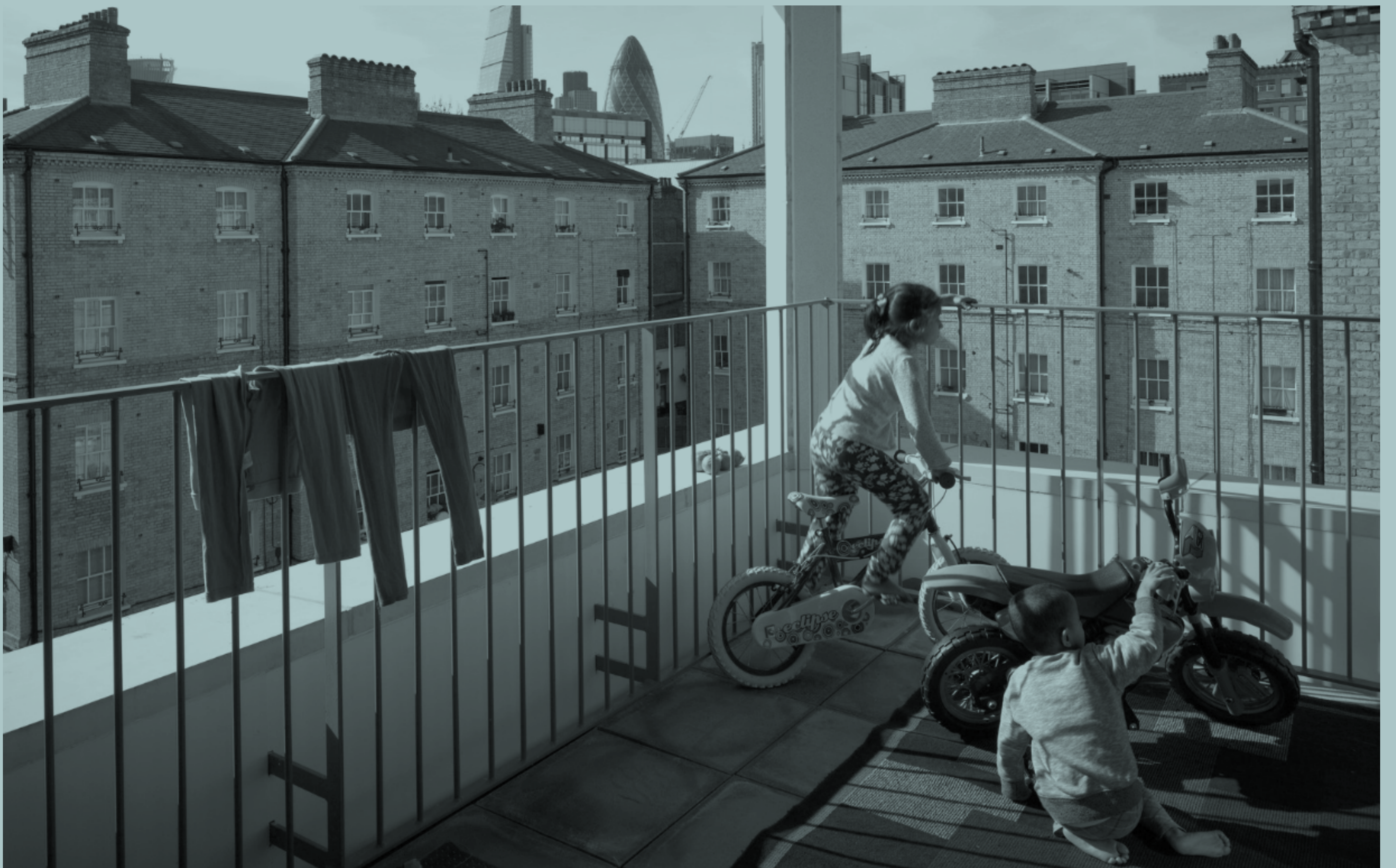
Darbishere Place, Whitechapel. Architects: Niall McLaughlin Architects. Photographer: Nick Cane.
